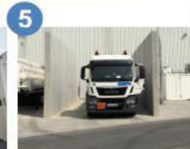
Grid injection plant
